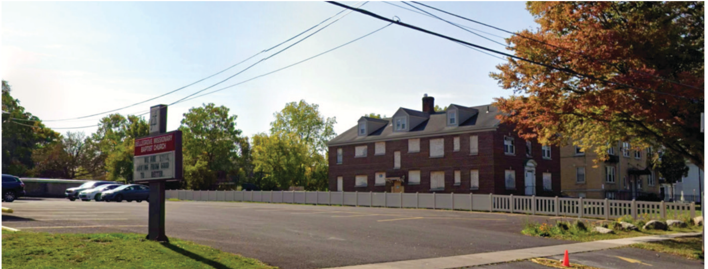
Completed Bellegrove Project: Porous Asphalt Parking Lot, Native Green Space, and New Fencing
