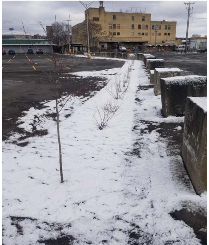
Completed Tree Trench at Evergreen Manufacturing
