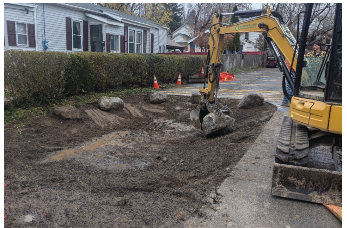
Construction of Rain Garden at 408 Lodi St
