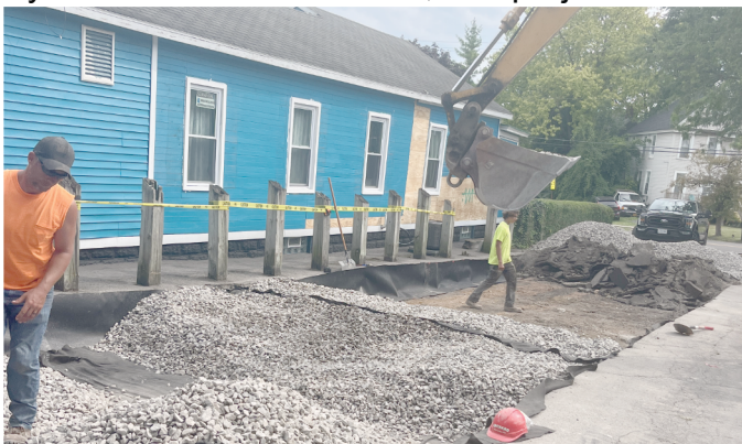
Construction of Porous Paving System at 414 Lodi St
