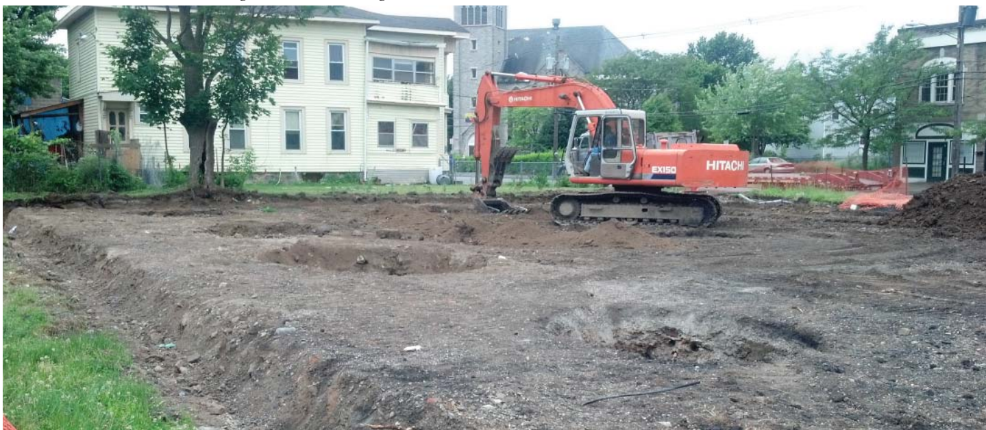
Save the Rain Vacant Lot Program - 701 Oswego Street under Construction
