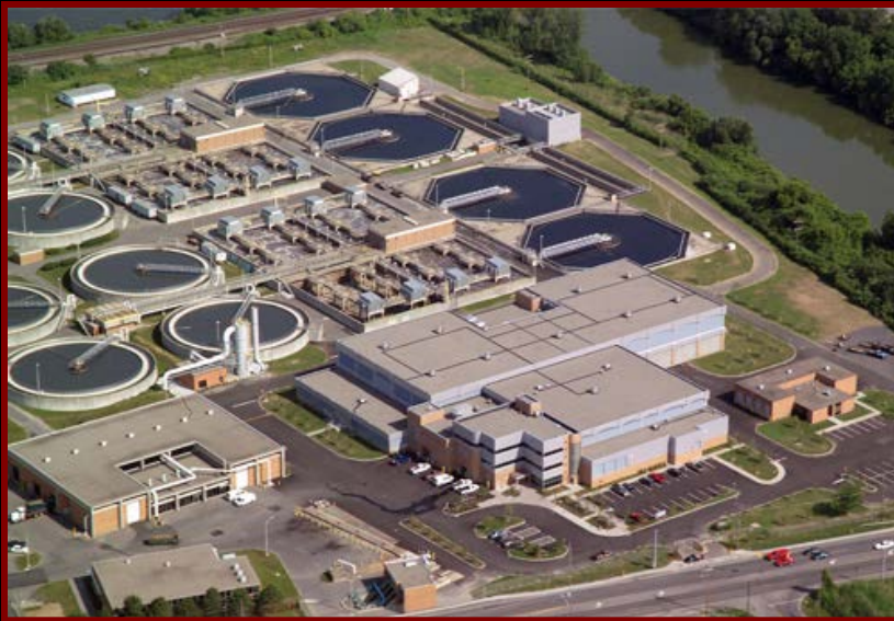
The Metropolitan Wastewater Treatment Plant (Metro)
