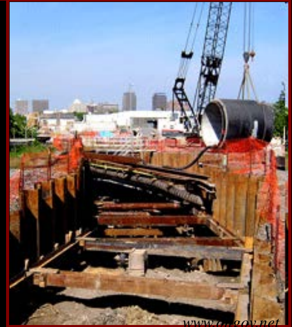
Installing the 144-inch pipe near Midland RTF (June 2006)
