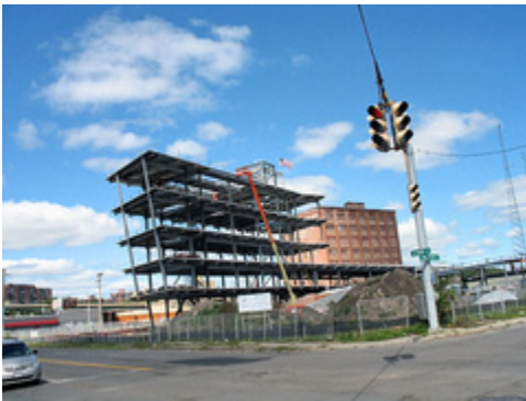
The SyracuseCoE headquarters building is being constructed on an old brownfield site
