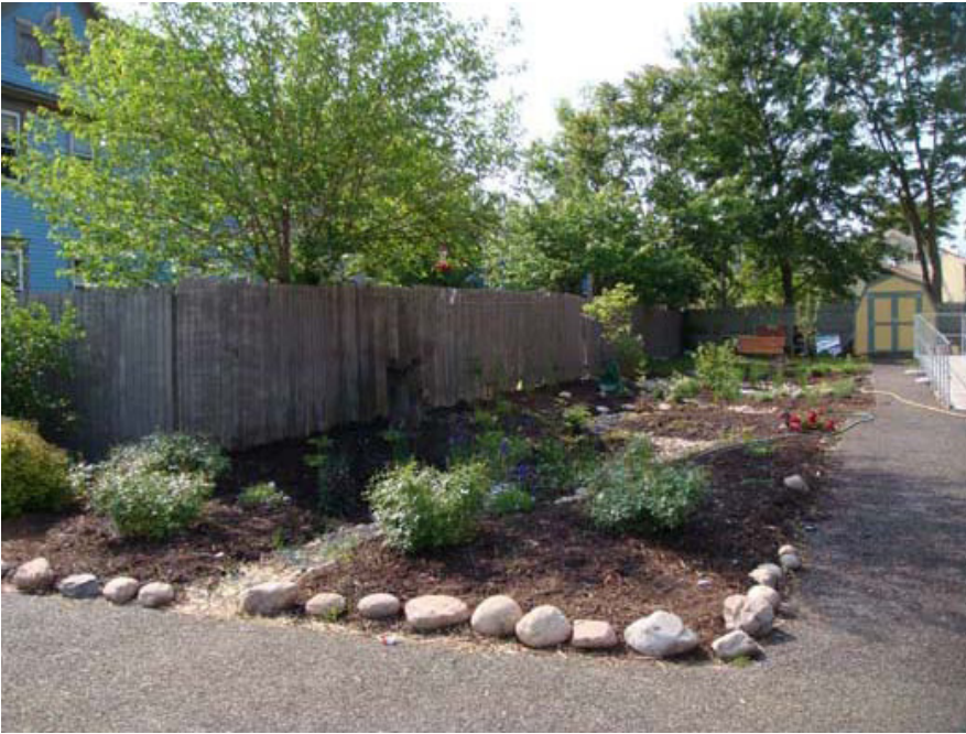
Roof runoff is directed into this rain garden at 515 Tully St.
