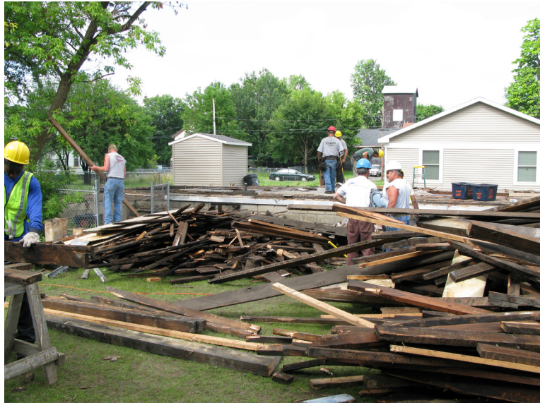
Above: Workers from Hope 4 Us Housing deconstruct a house on Syracuse's Near Westside.
