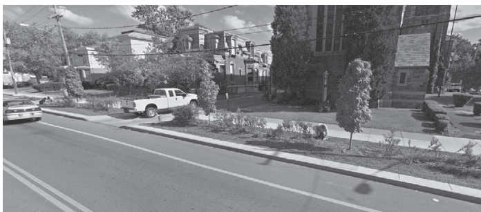
Project Joseph crew working on W Onondaga
