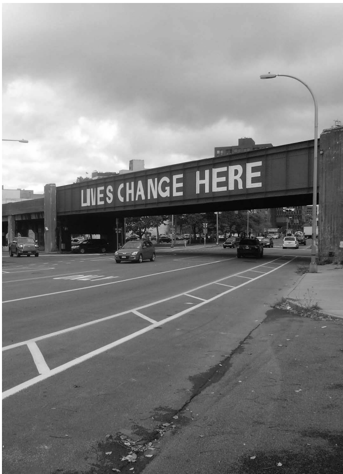
The rail bridge area near the Onondaga Creek
