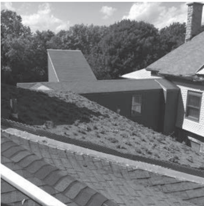
Upper Green Roof
